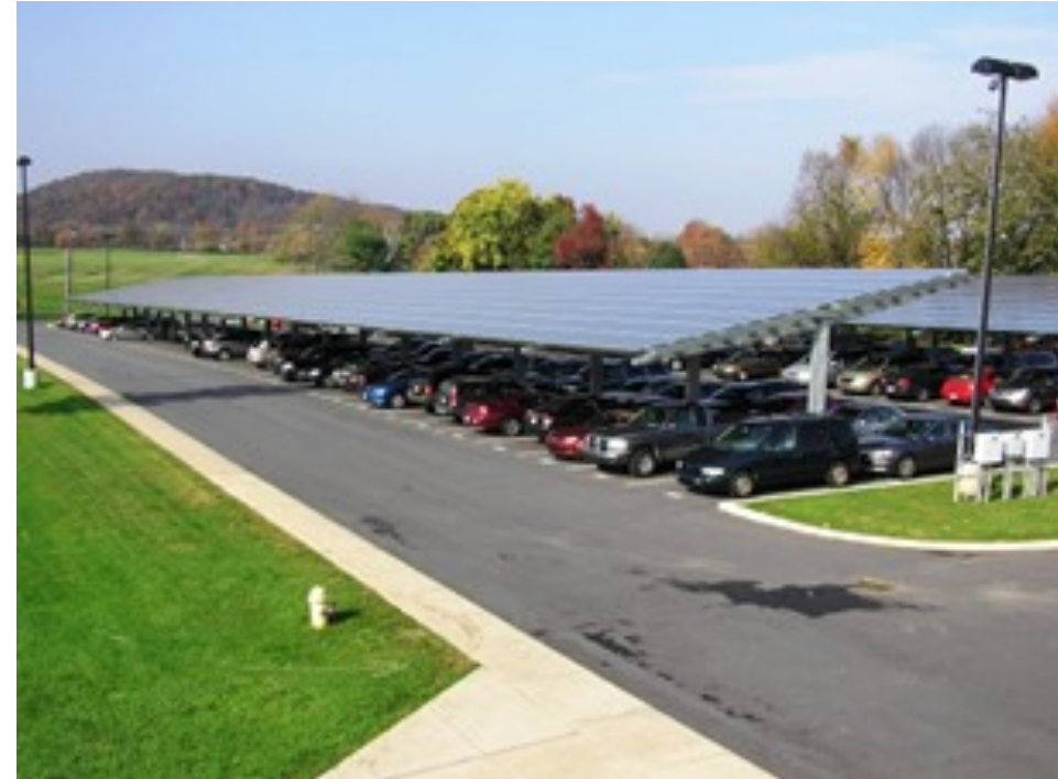
Solar Parking Canopy at Freedom High School
