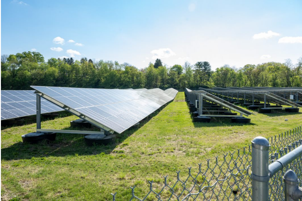
Typical ground mounting system with perimeter fencing
