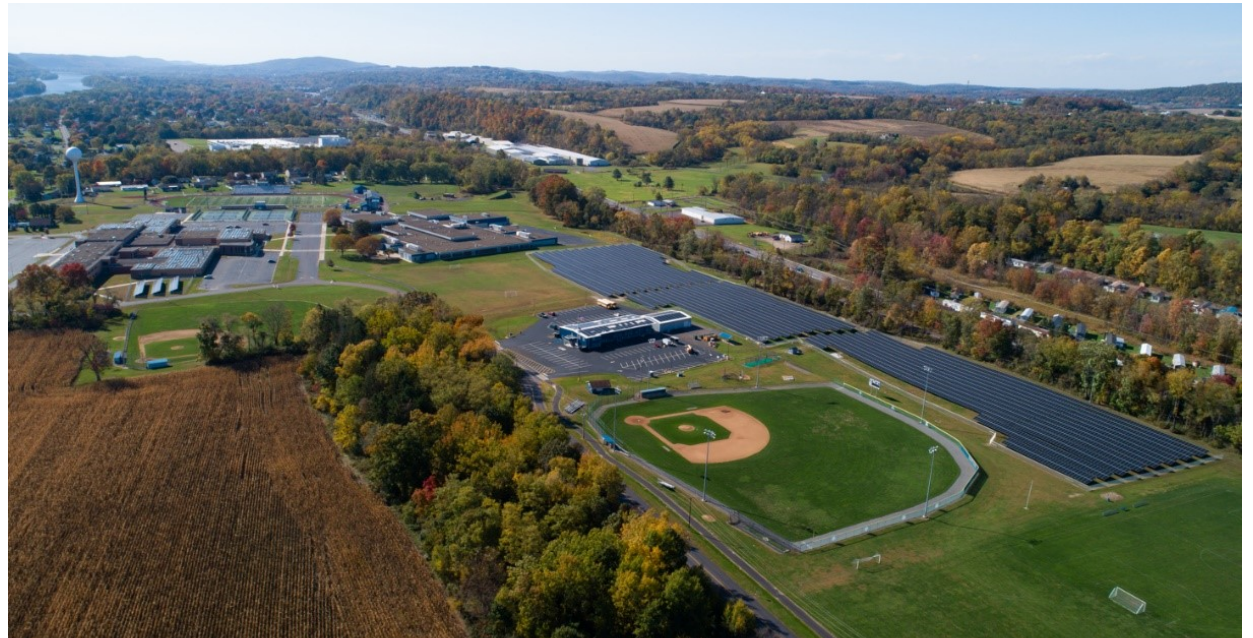
Central Columbia SD 3.8 MW Largest solar school system in PA !
