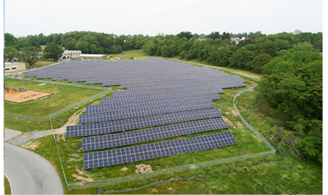
On settled landfill from flooding caused by Hurricane Agnes
